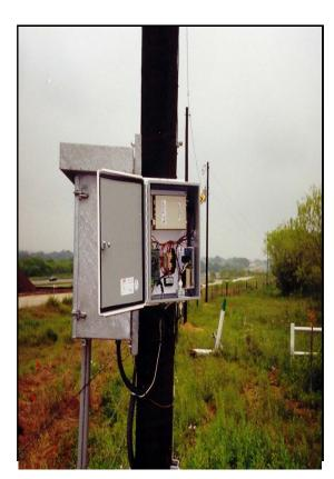
StarTrak Pigging Technologies, Inc. of Katy, Texas has developed master control monitoring stations that can communicate with satellite systems to provide operators with such capabilities as:
