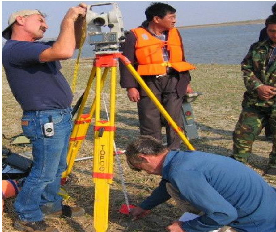
Preparation work being carried out- Northern China
